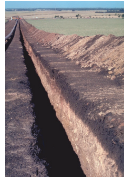
Trench section on the Lovely Banks Monocline slope showing shallower self mulching soil overlying highly calcareous subsoil
